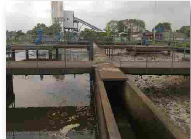
Wastewater treatment facilities
