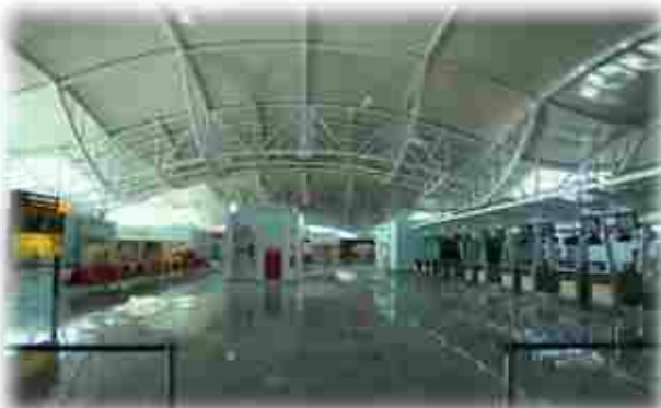
Skylight Concept Building
